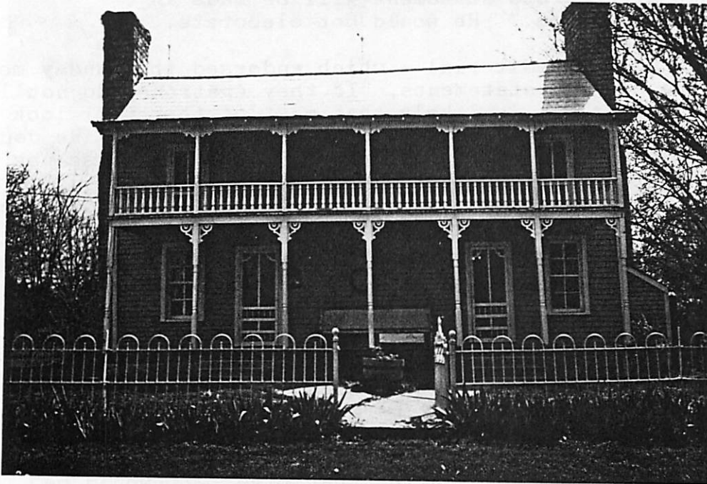
The Harris B. and Margaret C. Bradshaw Tuggle house, the main structure of which is log, was built ca. 1840 with major additions made by Britton and Lanna Thomas Litchford in 1920.
