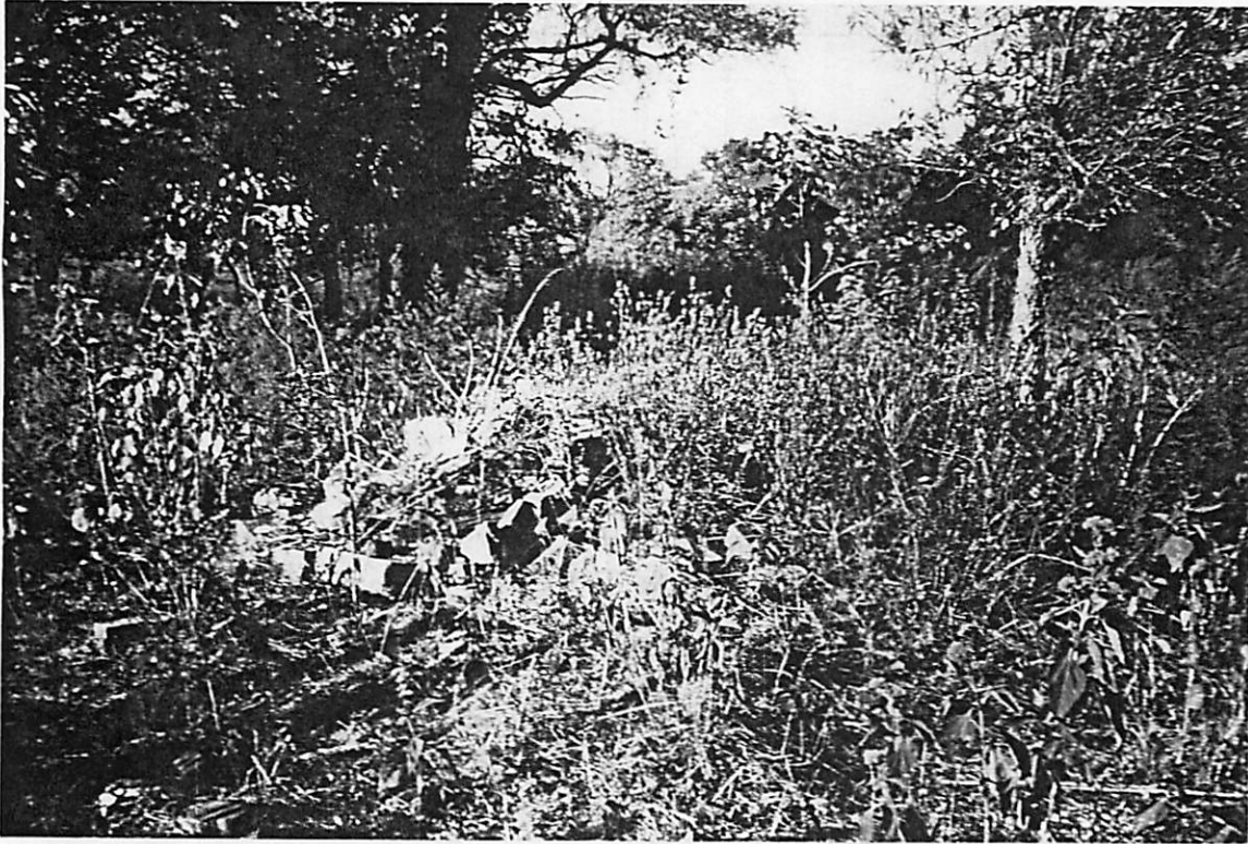
Foundation stones are all that remain of the spacious Josiah Rucks house built in 1820.
