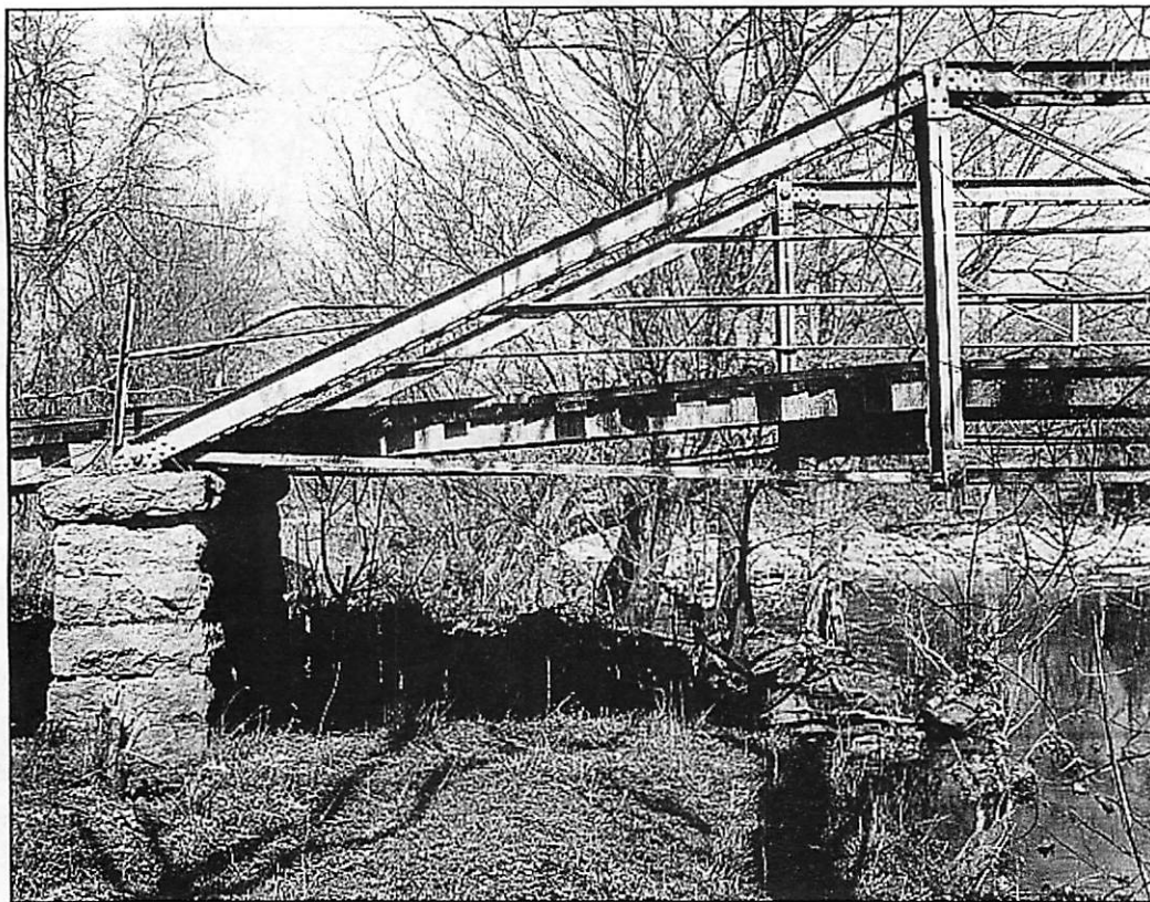
Figure 10. View of west end, hip panel, looking north (1985 HAER photo).
