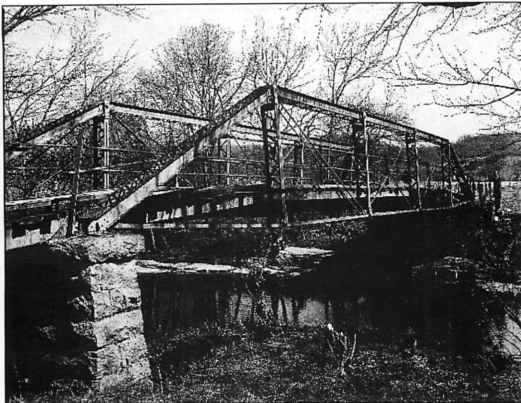
Figure 9. View of bottom chord, looking east (1985 HAER photo).
