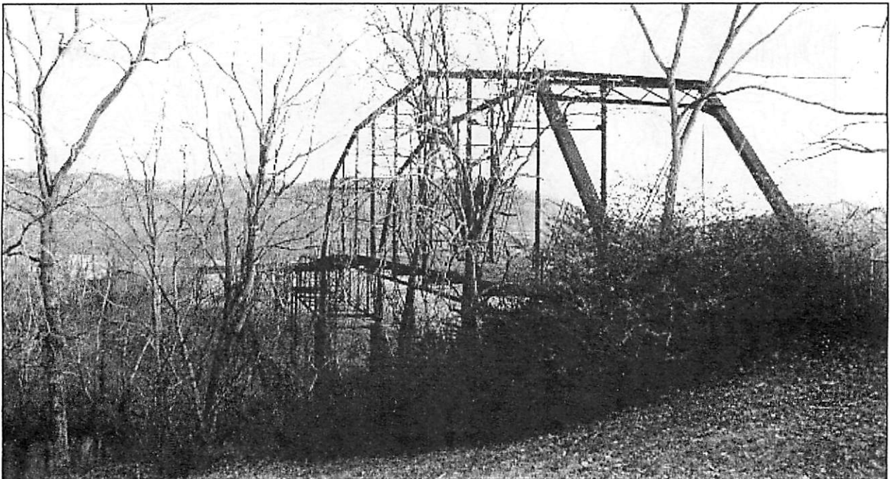
Figure 3. The now closed Stonewall Bridge facing east. An unusual – and particularly dangerous – feature was the 90 degree curve in the bridge’s approach ramp on the opposing eastern bank.
