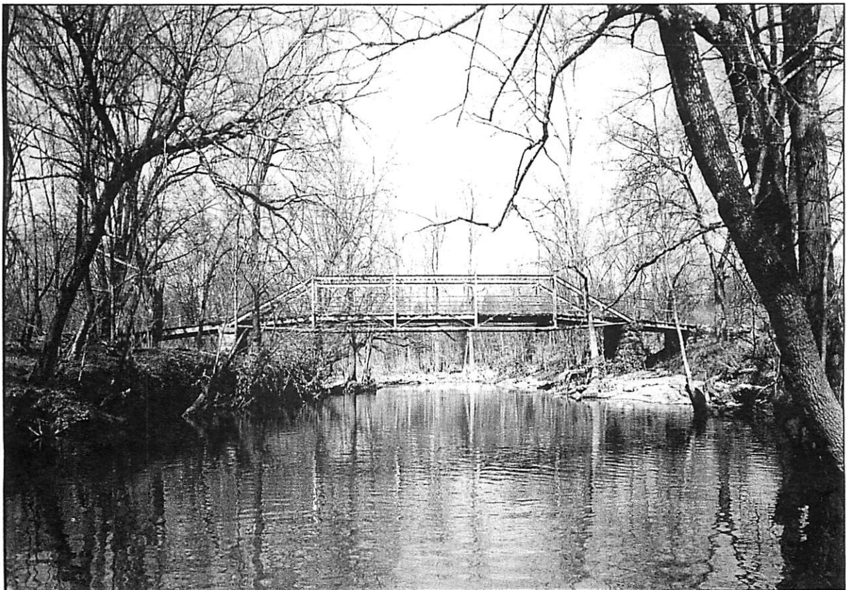
Figure 6. View of south elevation, looking north (1985 HAER photo).
