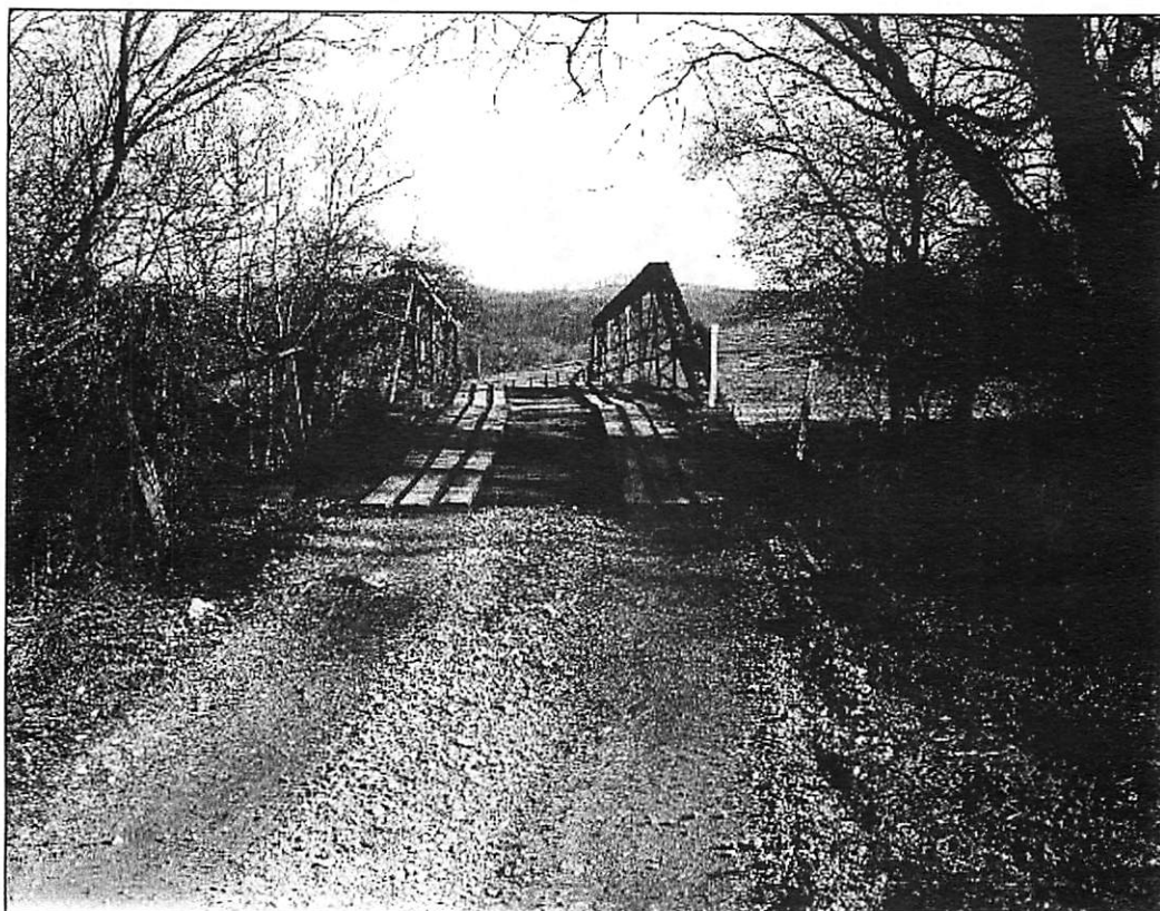
Figure 7. Through view of bridge, looking east (1985 HAER photo).
