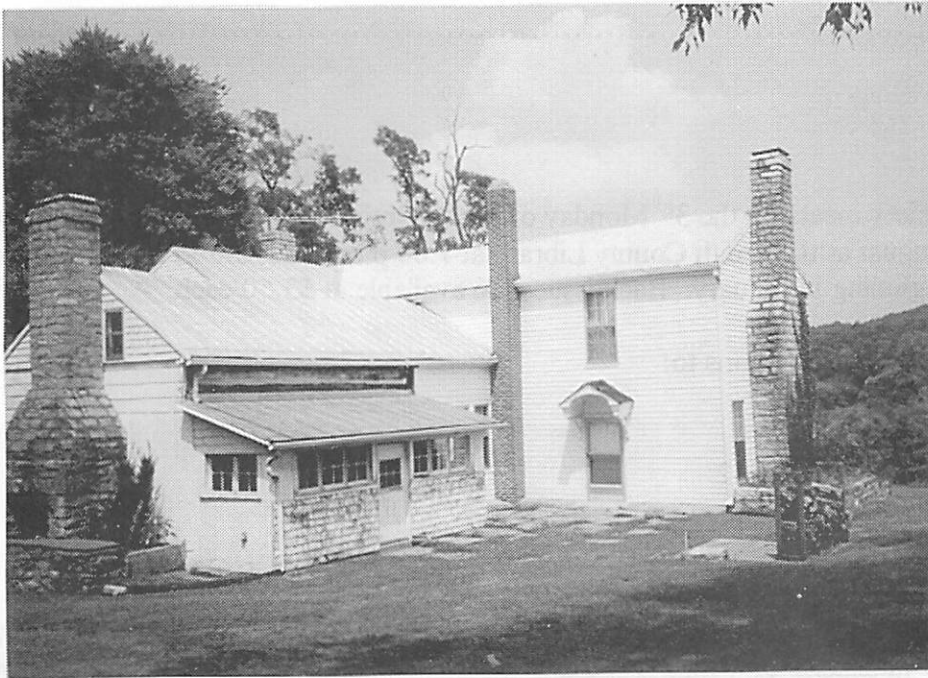
THE BACK OF CHEERY HEIGHTS SHOWING THE TWO-STORY KITCHEN
